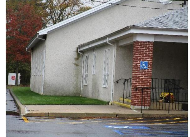
Rain gardens can be installed in the turfgrass area near the entrances of the building to capture, treat, and infiltrate stormwater runoff from the roof. Planter boxes can be placed under downspouts where there is not enough room to install a rain garden. A preliminary soil assessment suggests that the soils have suitable drainage characteristics for green infrastructure.
